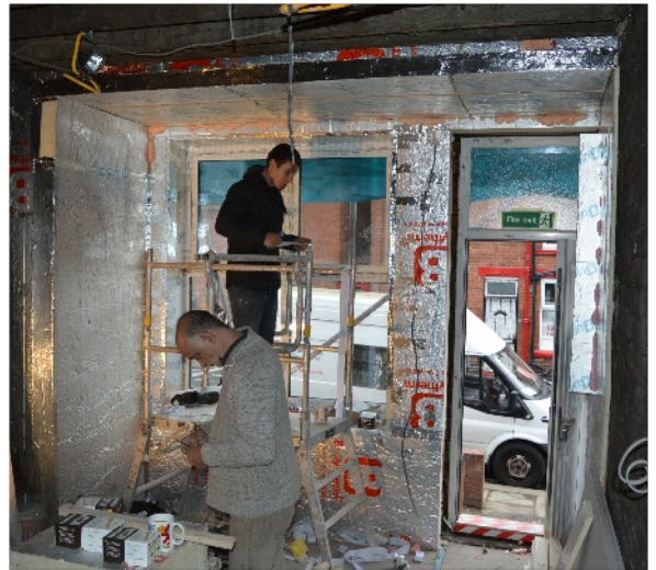
The front room of a terraced house before and after internal wall insulation is fitted
