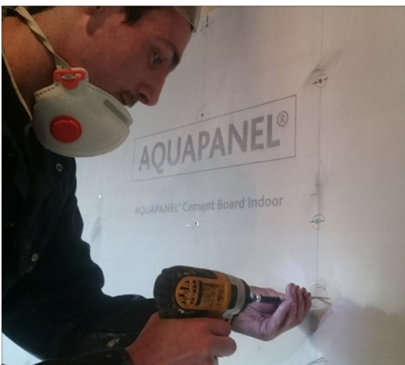
Fitting board to the internal insulation ready for plastering
