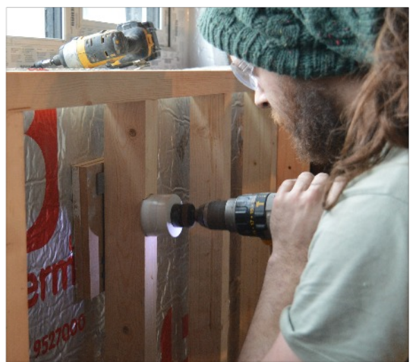
Building a frame over the insulation board
